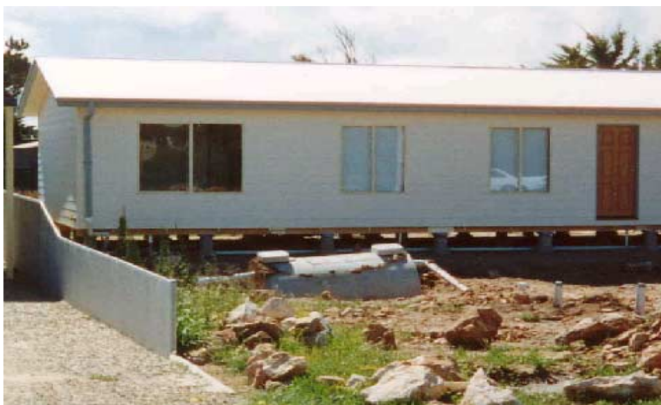
Take note: Concrete tanks can float!
