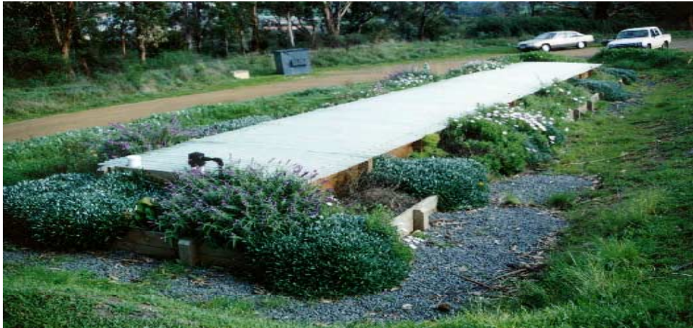
Photo: Above ground Modified Adsorption Trench (elevated)-MAT(E) Kingston Golf Course, Tasmania
