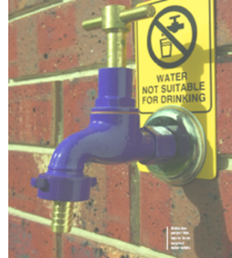
Figure 4: Outdoor Tap and Labelling
